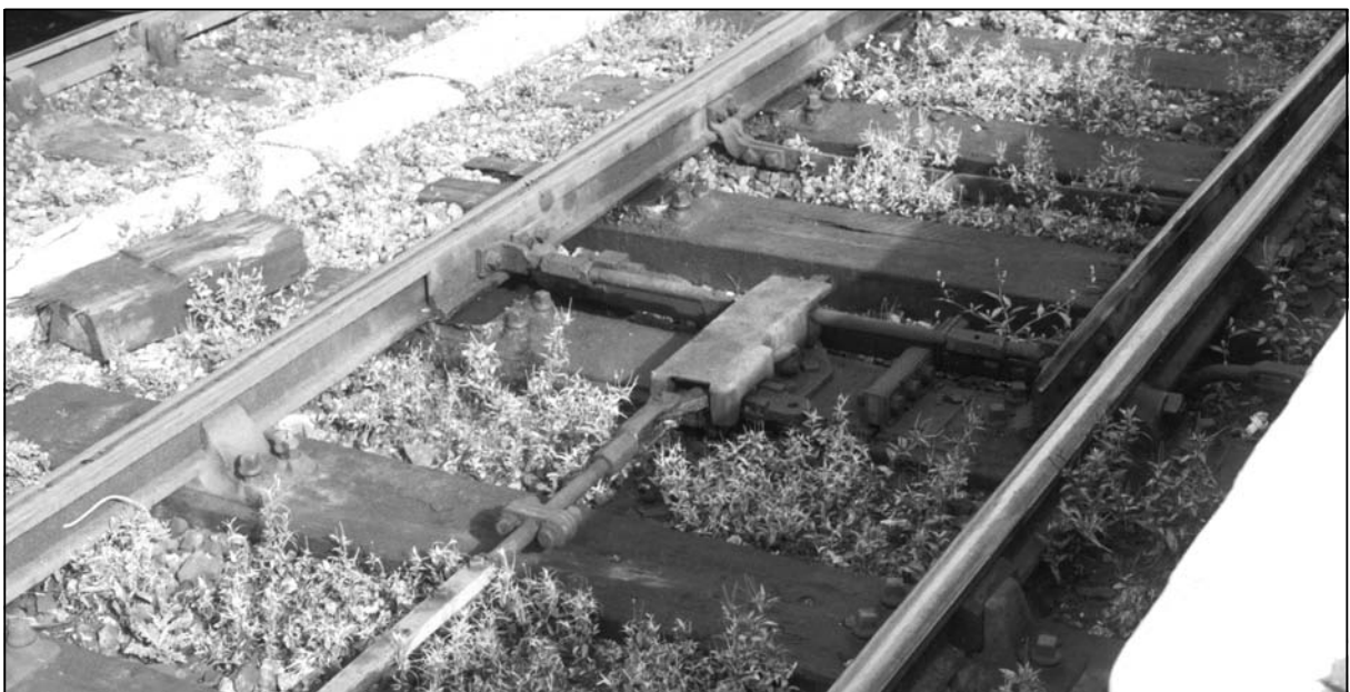
Photo 2.35 GWR style front stretcher with facing point lock. Under the cover the centre has a flat section notched to receive the locking bolt. The second stretcher, just visible beyond the sleeper, is a flat bar.
