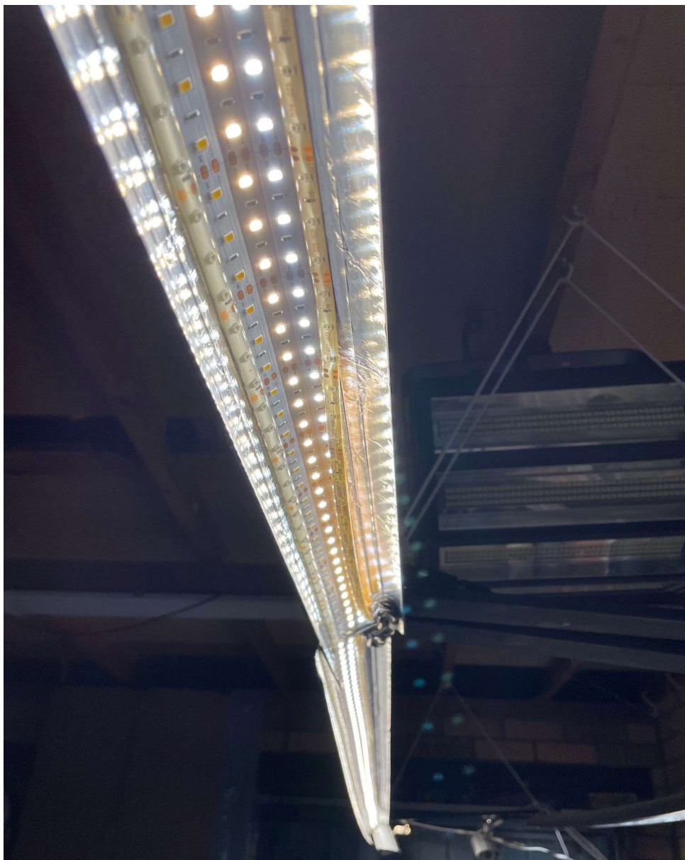
A lighting gutter showing different colour temperature strips
