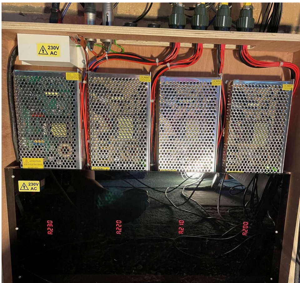
High current 12V power supplies and associated dimmers behind perspex panel at bottom.
